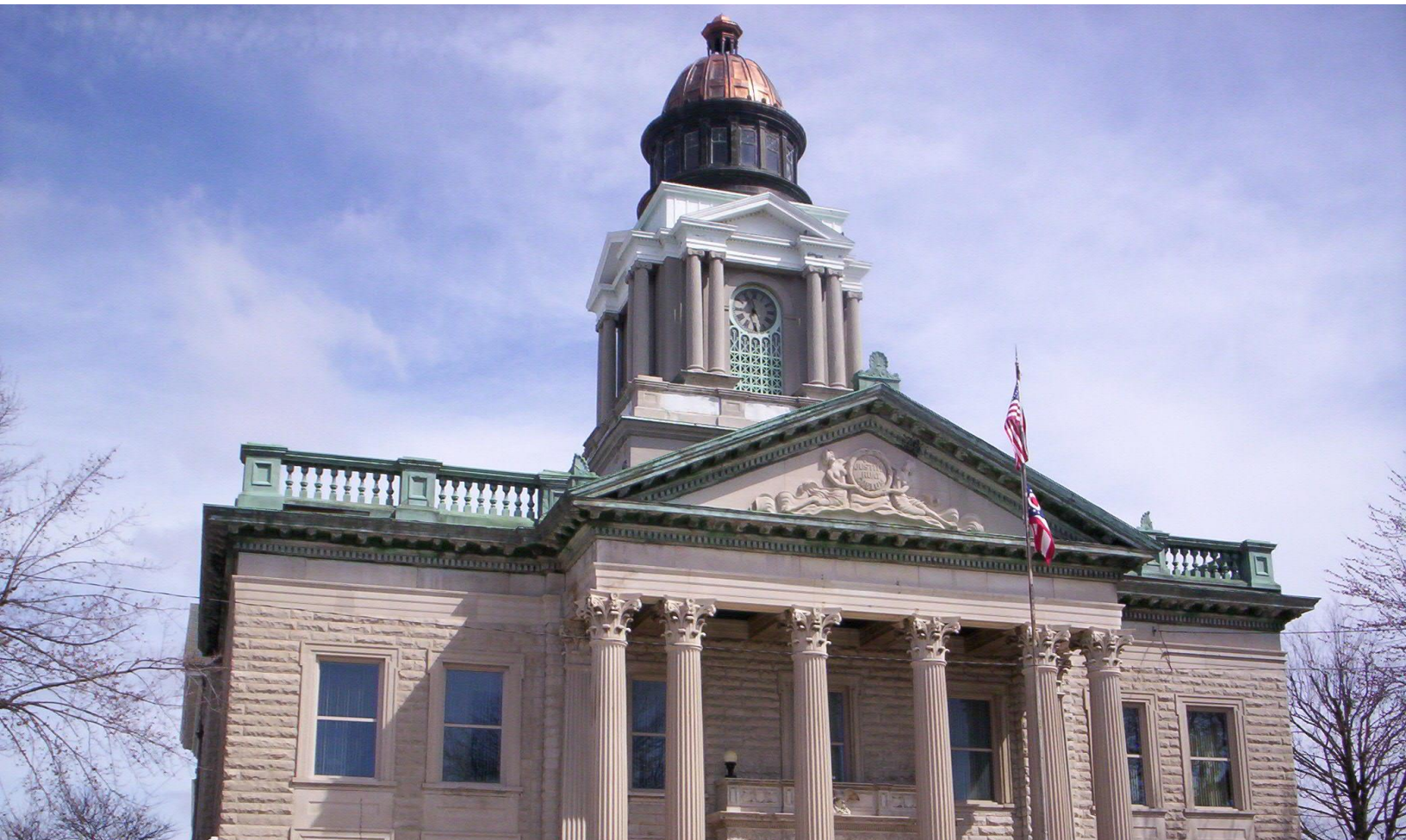
Crawford County Courthouse Bucyrus, Ohio
